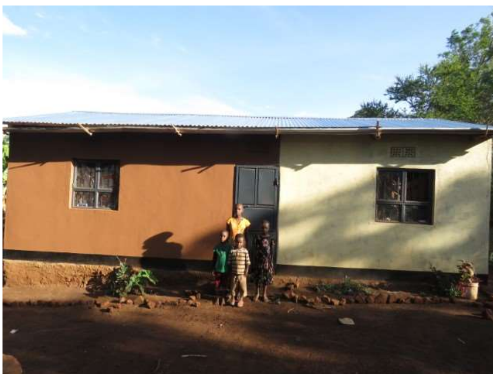
These children live with their parents. The parents had started building a house but could not finish it but because of financial problems, they lived in that unfinished house. Now that the church has helped them finish it, they live in a nice safe house.
