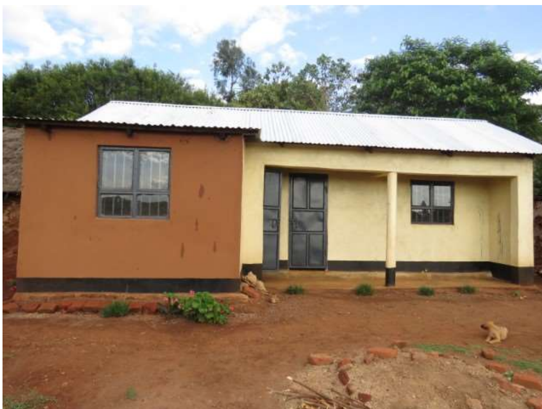
Beneficiary number TZ061200098 lives with her grandmother. The grandmother gave the piece of land to the beneficiary. They lived in a mud house with their animals. The house was very poor such that a hyena ate a goat sometimes ago. It was leaky and they were not safe at all when it rained. The new house has given them new hope and joy.
