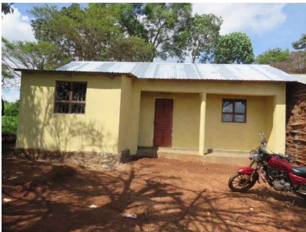
One of the houses at TZ0612 completed and ready for the family to move in. All the houses were built with three bedrooms and a sitting room.
