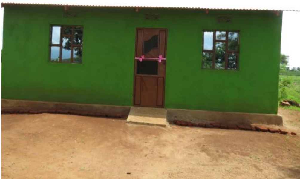
A completed house at TZ0275. The families are so happy.
