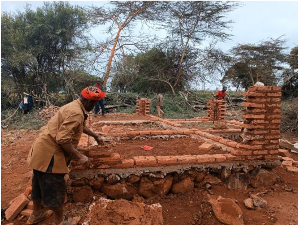
The beginning of the construction at TZ0163. A mason continues with the construction of the wall upwards.
