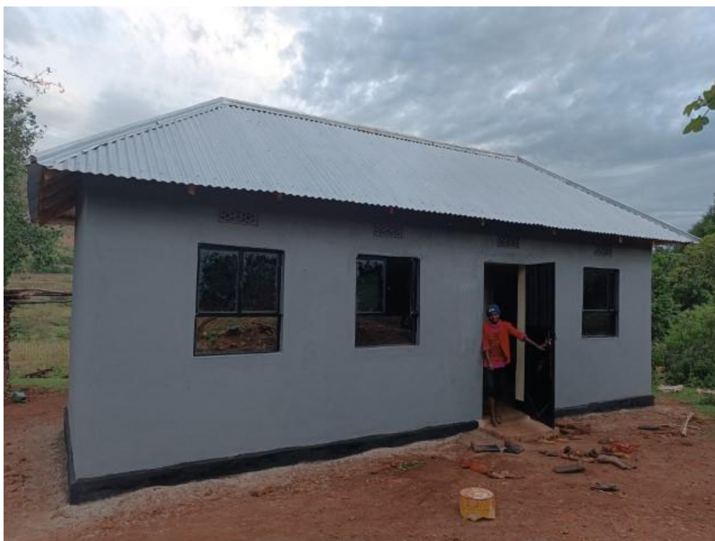
A house at TZ0163 is completed by being roofed, painted and glazed, ready to use.
