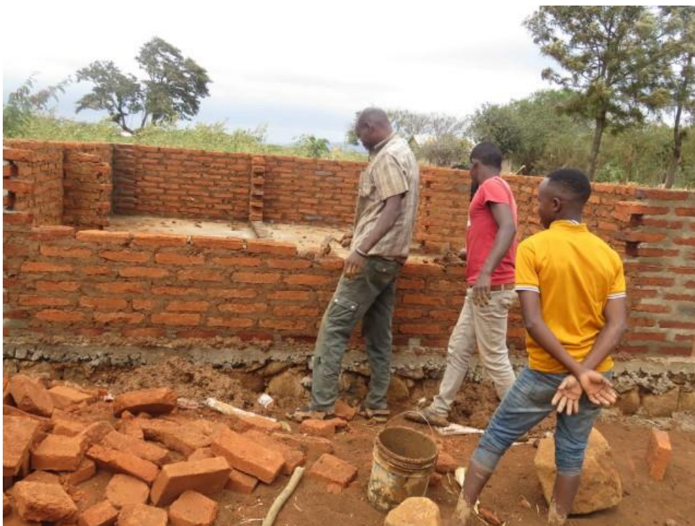
The construction of a house at TZ0275.
