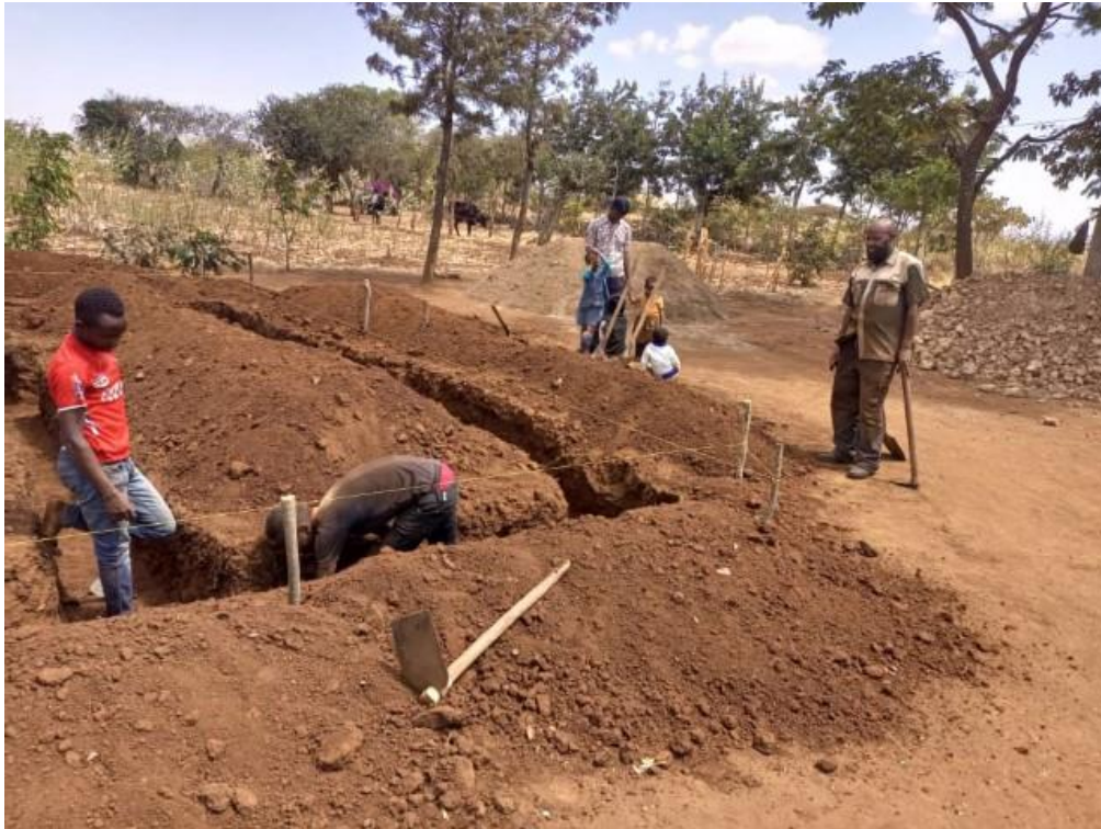
Early stage of the house construction. Laborer are digging the foundation of the house.
