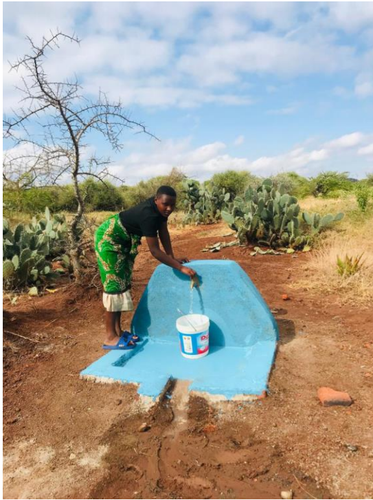
A community A hand washing outletwater
