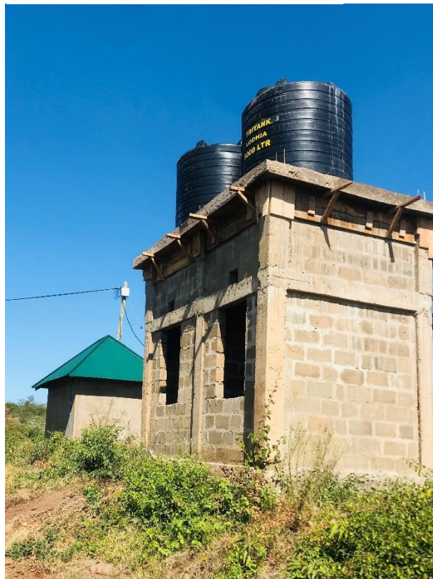
A water tower.
