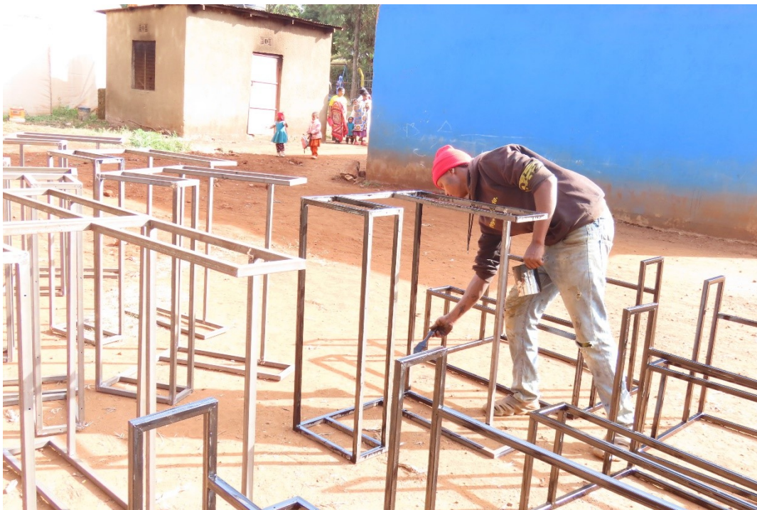
The photo shows the painter painting the steel to make it look good but also to prevent it from rusting.
