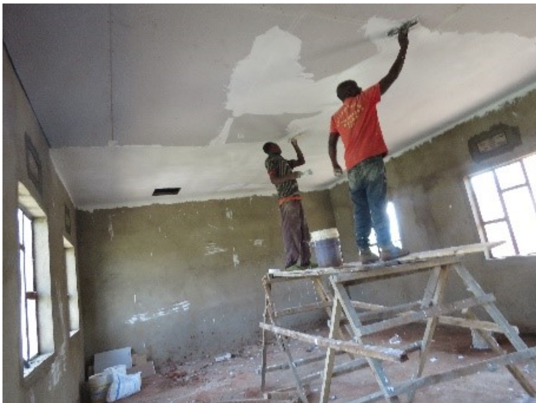
The next picture is painting on the gypsum board which built in both classes.
