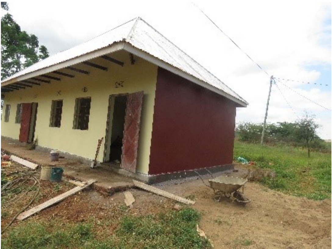
The finishing of the classrooms proceeding and here it is at the stage of painting outside and inside the classrooms.
