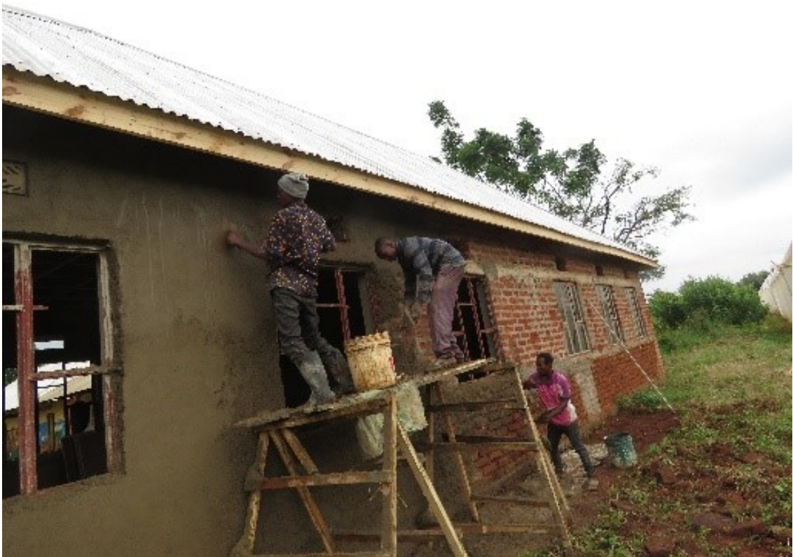
This photo shows the builders who have already started the finishing work of the classrooms and here they are plastering and the second photo the technicians are closing the draft for the gypsum board.
