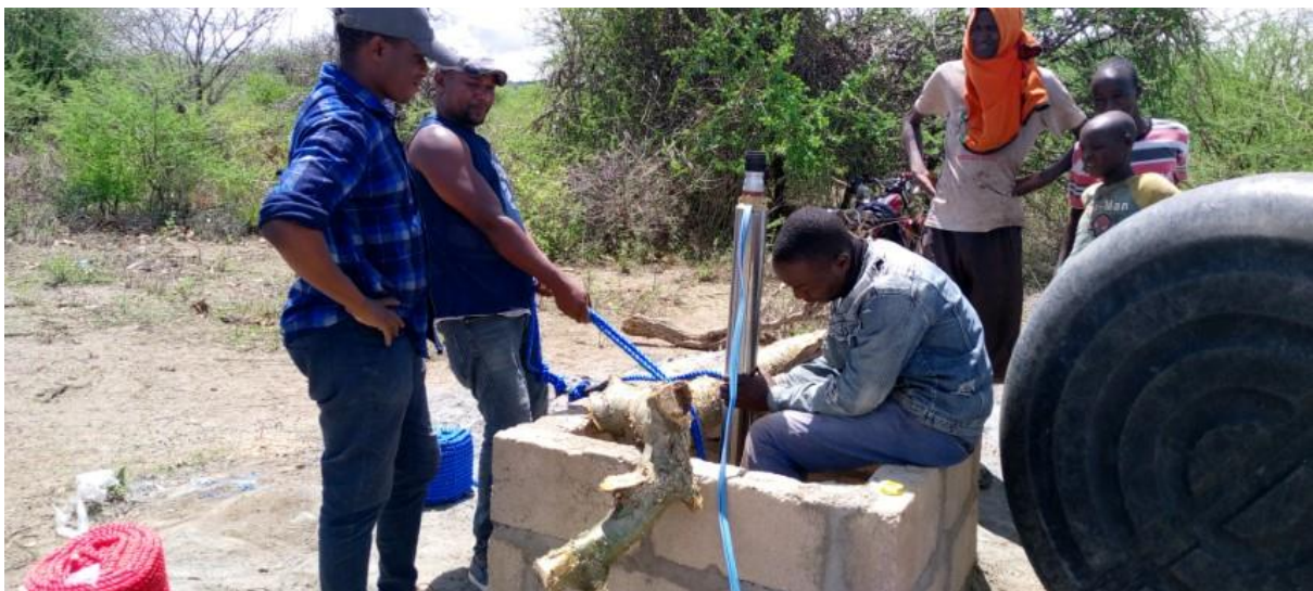
Water engineers loading down a water pump as installation down the bore hall to pump water from the hole to the reserve tanks for project consumption.
