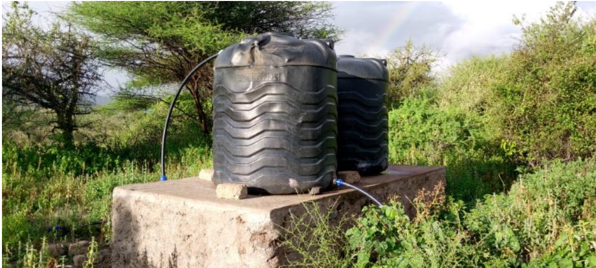
Water tanks as reserve of water from the borehole ready to be transferred to the water tapes for participant and the community uses at the project center.
