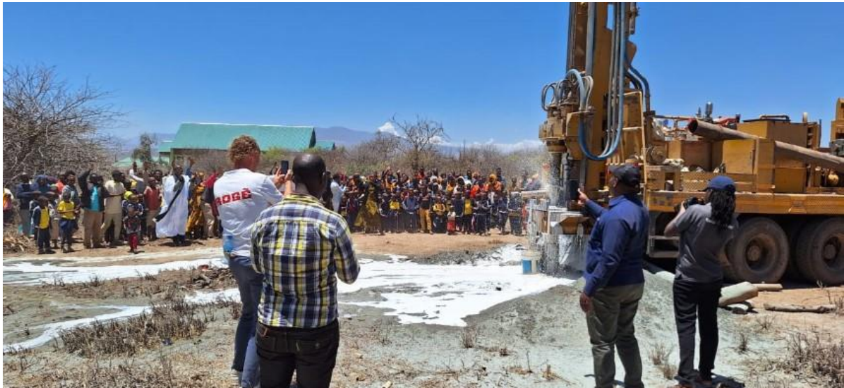
Drilling in progress and already found underground water at a distance of 80 mtrs down as the first step with dirty and muddy mixed with water from the borehole.
