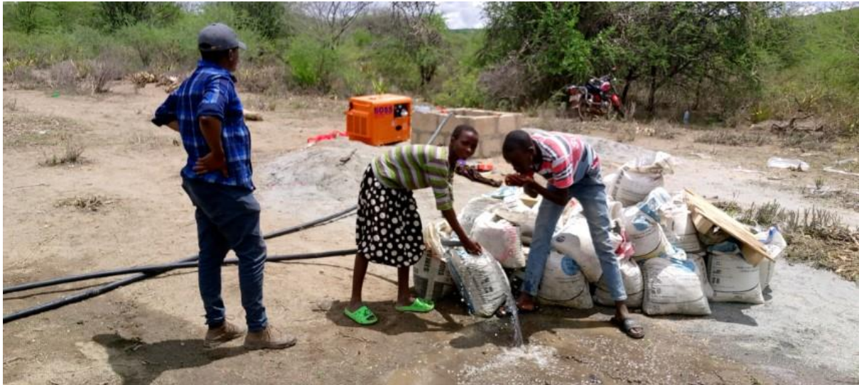
Church members testing and enjoying water pumped from the borehole by washing faces and flashed the away with joy while testing the water volume per hour from the well and its pressure vertically and lateral.
