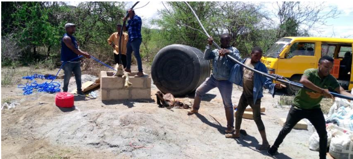
Water engineers seeping down a water pipe to pressure and final clean water from the borehole for pressure test and water volume to finally be consumed at the project center.
