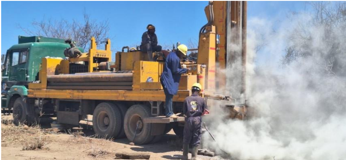
Drilling machines at the drilling point at the church clearing ground ready to start drilling a borehole.
