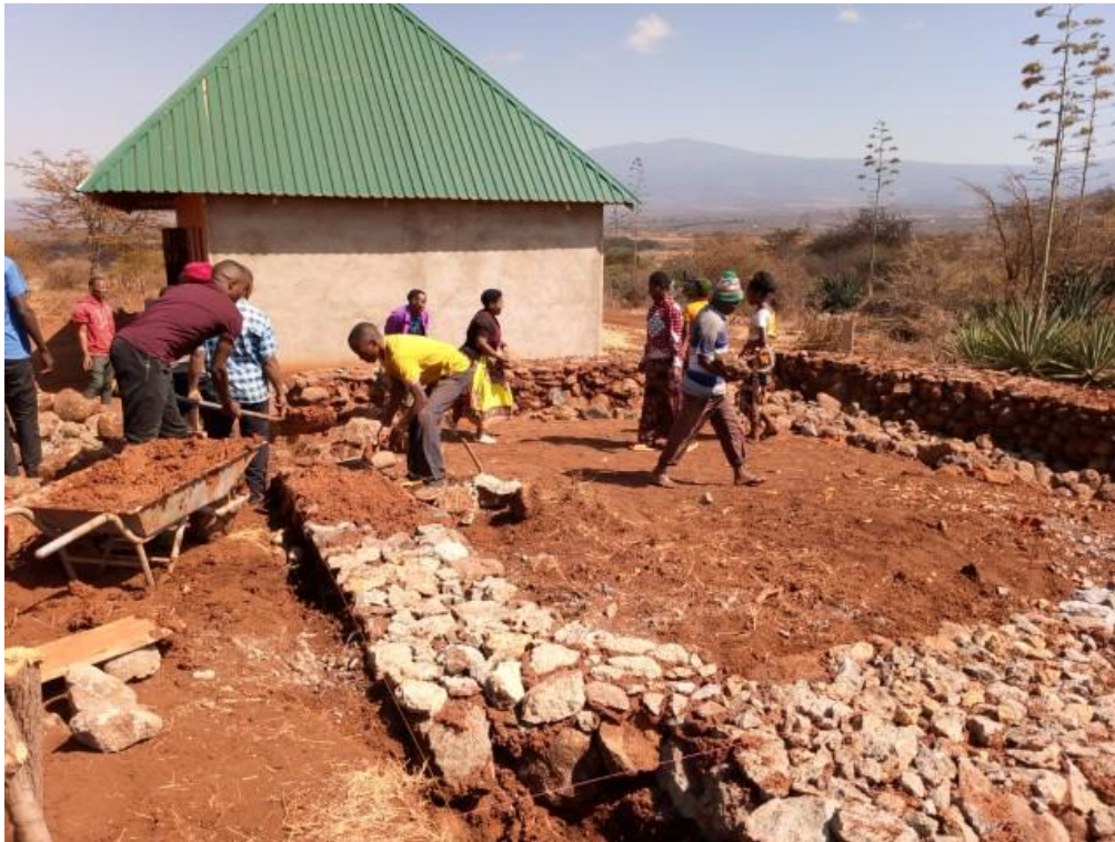
Parents/caregivers, church members, technicians and the child ministry team mobilized each other to construct the foundation for three classrooms.
