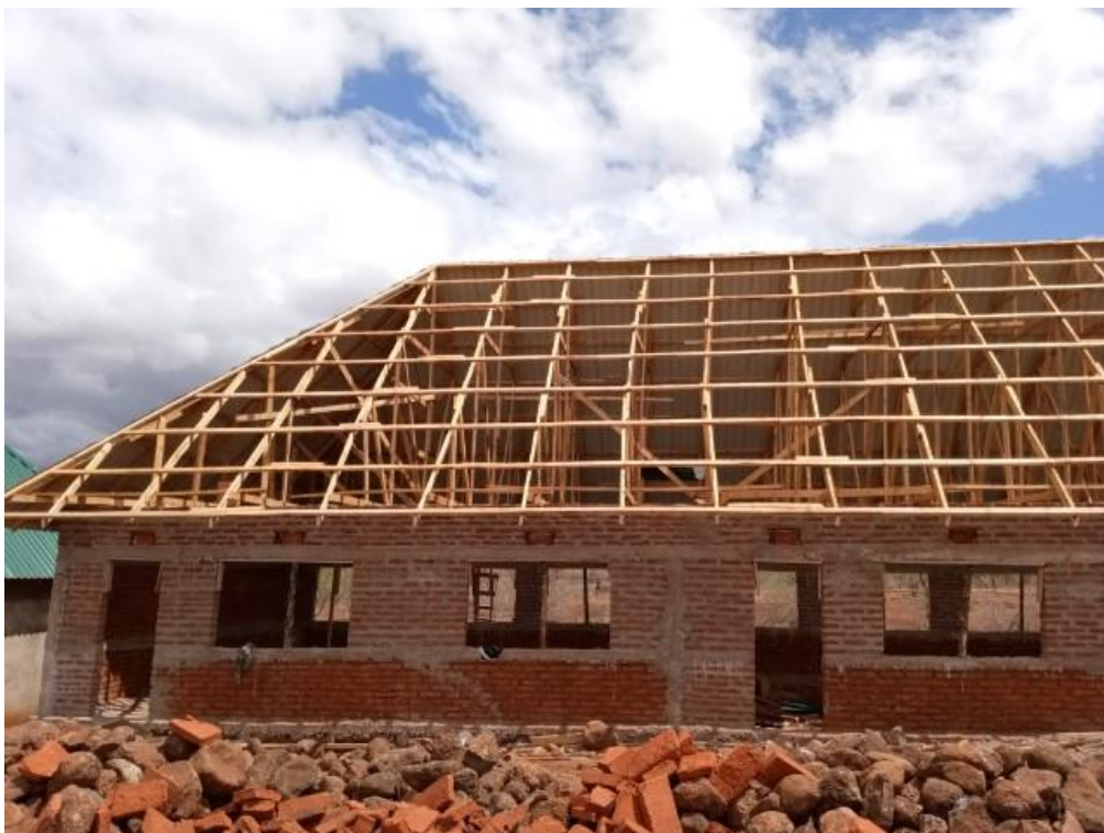
The technicians are now fixing iron sheets to complete the roofing stage.
