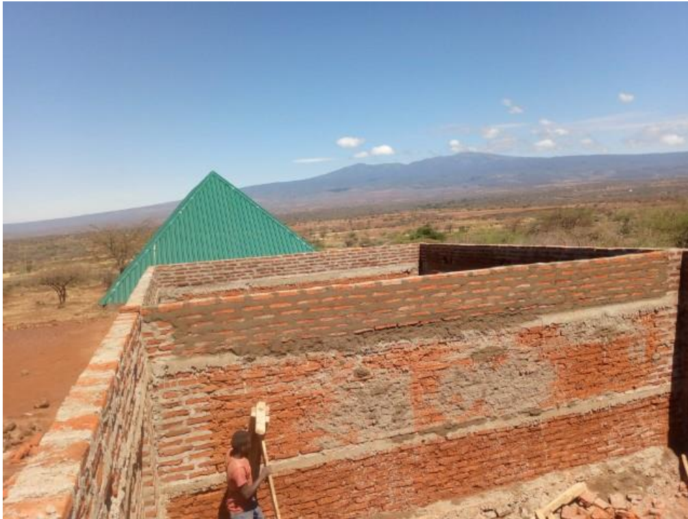
The completed wall of the three classrooms.
