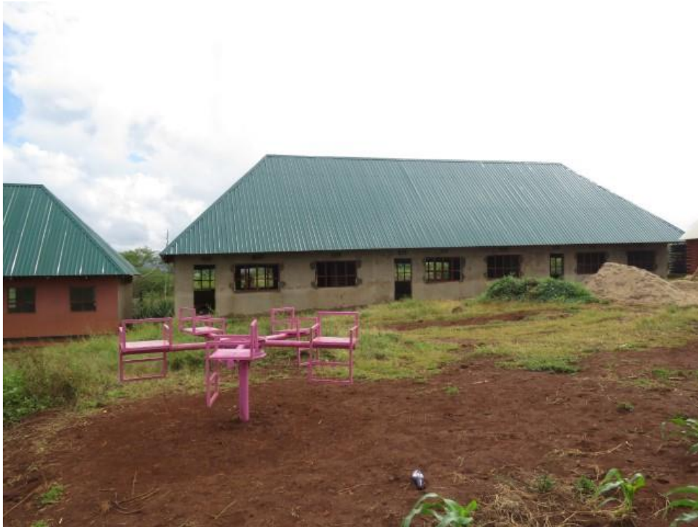
The third stage of the construction: fixing windows and doors, plastering inside and outside the classrooms.
