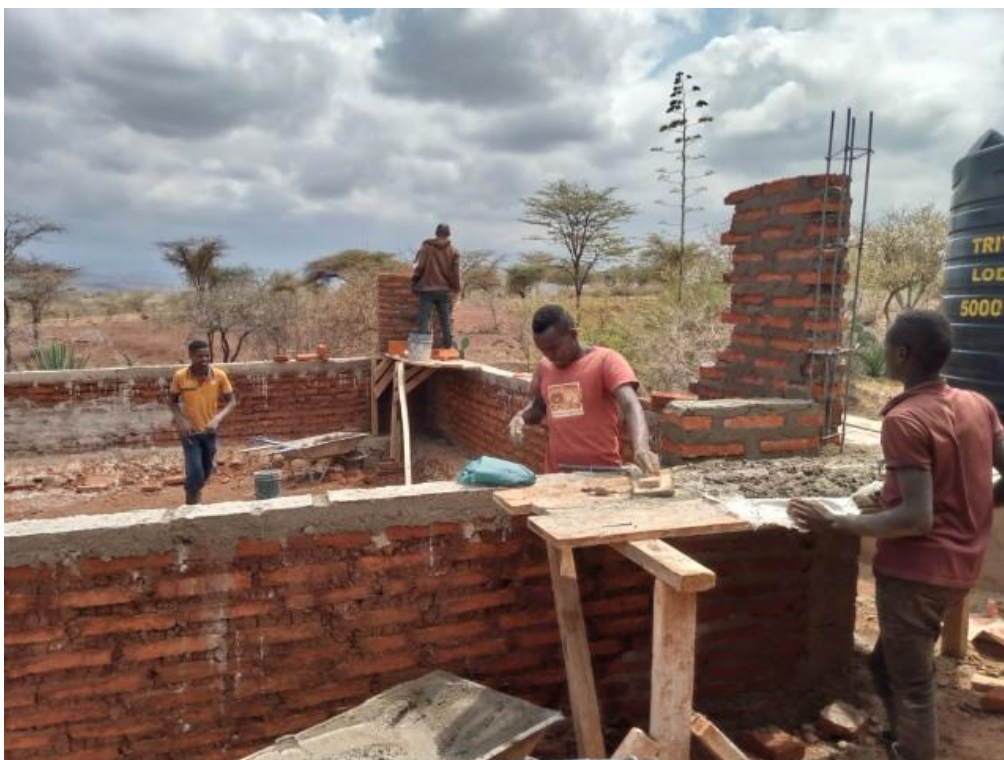
Technicians are constructing the walls after concreting the slab and the foundation.
