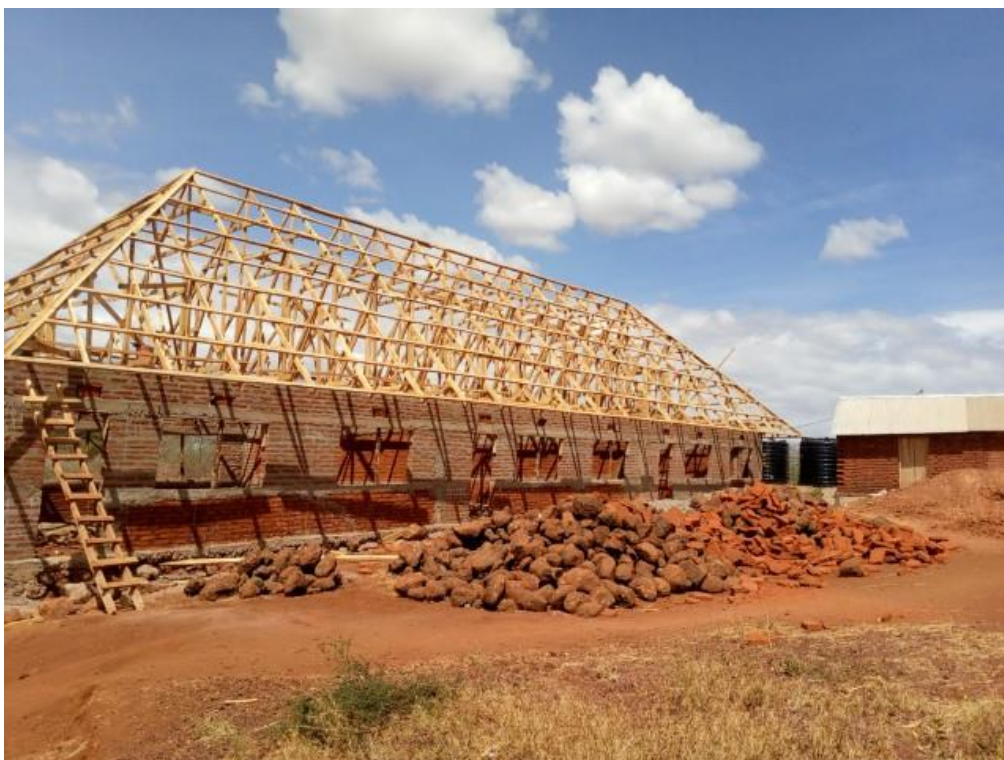
The completed carpentry work during roofing stage.
