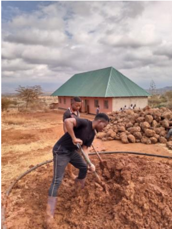
The project director and a church member while admixing mud for the foundation of the building. Church has been mobilized to participate and give their full potential to accomplish the task.
